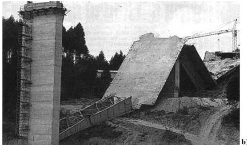
Figure 1 Spectacular accidents have motivated the community to improve safety: a) the Aloha Airlines flight 243, April 29, 1988, due to corrosion insufficiently controlled by maintenance; b) the Injaka bridge collapse, July 1998, due to a poorly controlled construction process
