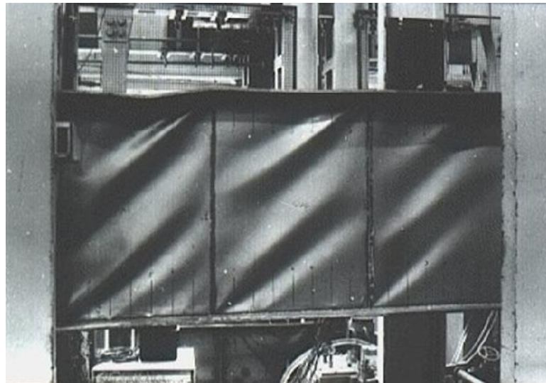
Figure 3.7: Examples of shear buckling
