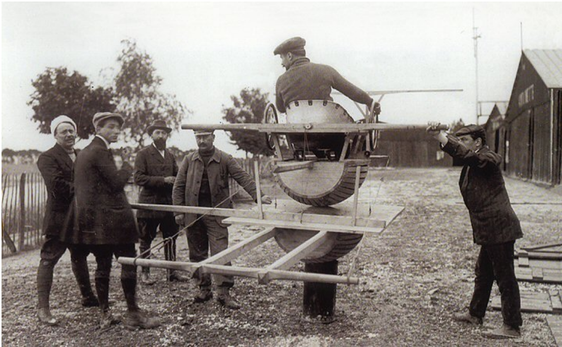
Figure 1.7 – Pilot training with “tonneau antoinette” at levavasseur’s workshop in 1910
